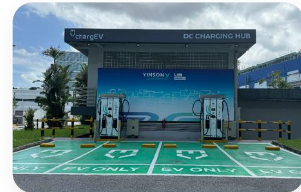
Vehicle Park with EV Charging Stations
