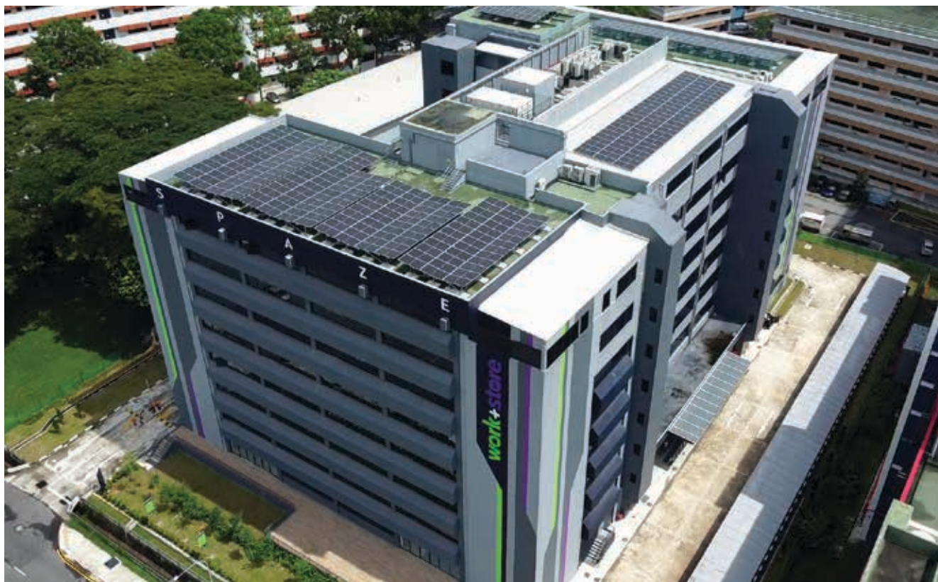
Solar panels on the rooftop of 202 Kallang Bahru
